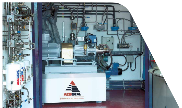
Extensive AESSEAL® test facilities
